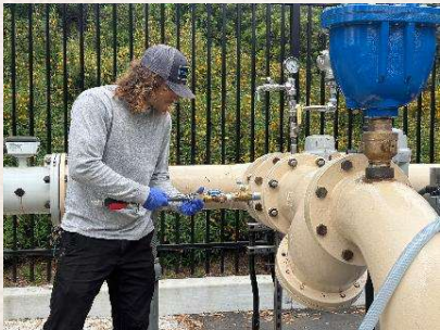
Installing the quill
