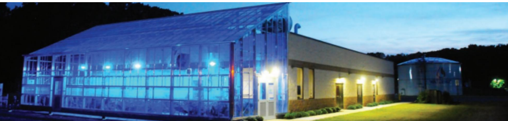
WaterHub's greenhouse, administrative building, and reclaimed water storage tank at Philip Morris USA in Richmond, VA [Photo credit: Sustainable Water]
