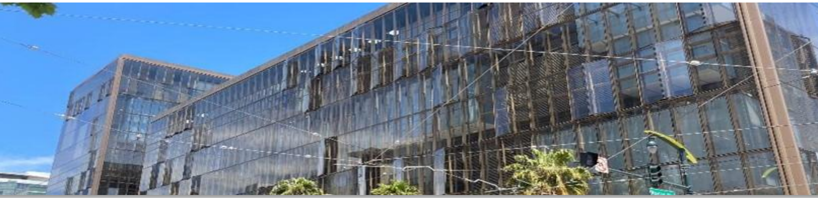
Uber's headquarters in San Francisco is recycling its graywater onsite [Photo credit: HTEC]
