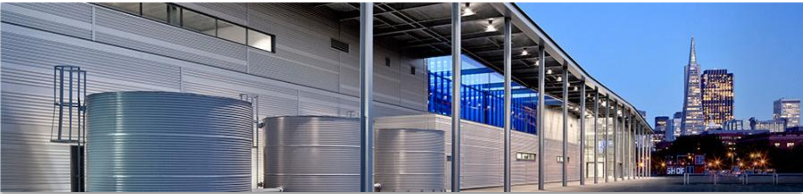
Pier 27's rainwater tanks in San Francisco, CA [Photo credit: Port of San Francisco]
