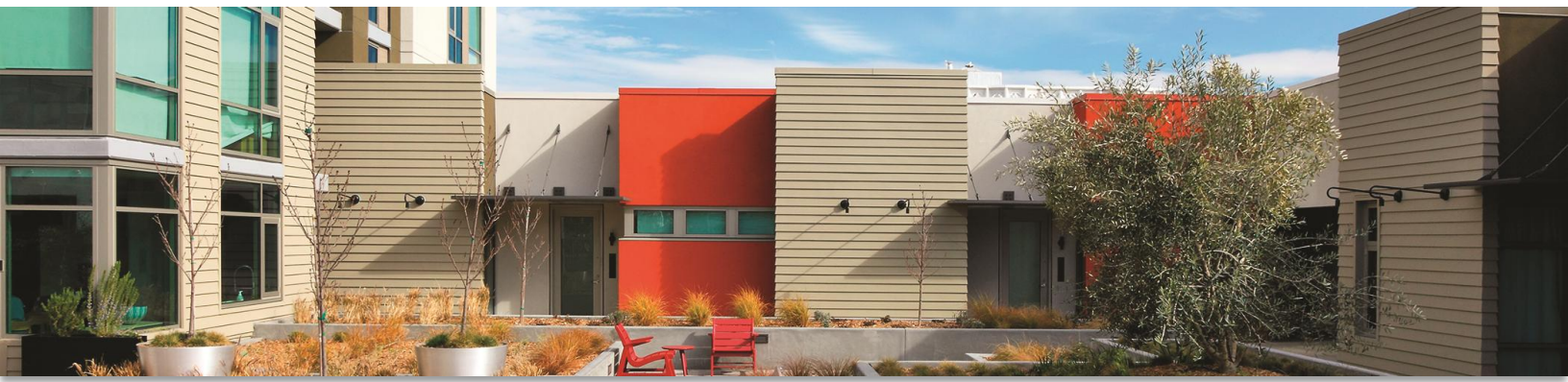
38 Dolores courtyard in San Francisco, CA, that is capturing rainwater for irrigation [Photo credit: BAR Architects]
