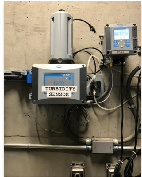
FIGURE 9.1: Example of a turbidity sensor [Photo credit: San Francisco Public Utilities Commission. No public source. Permission to use.]
