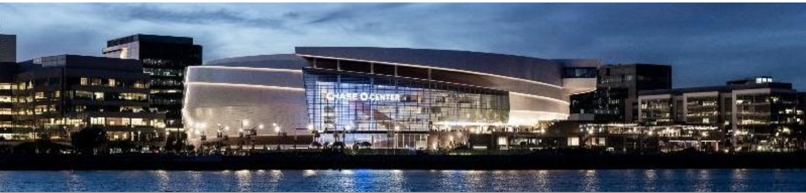
Chase Center in San Francisco, which is an ONWS [Photo credit: Chase Center]
