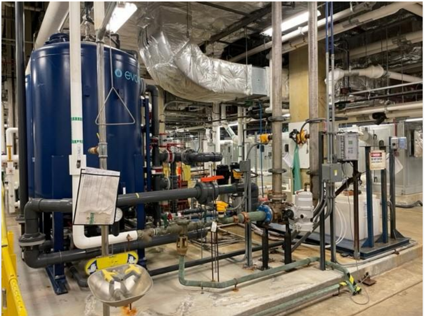
The National Museum of African American History and Culture Building features a rainwater harvesting system [Photo credit: San Francisco Public Utilities Commission. Permission to Use.]
