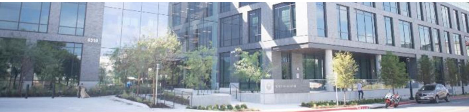
City of Austin Permitting and Development Center [Photo credit: Austin Water]
