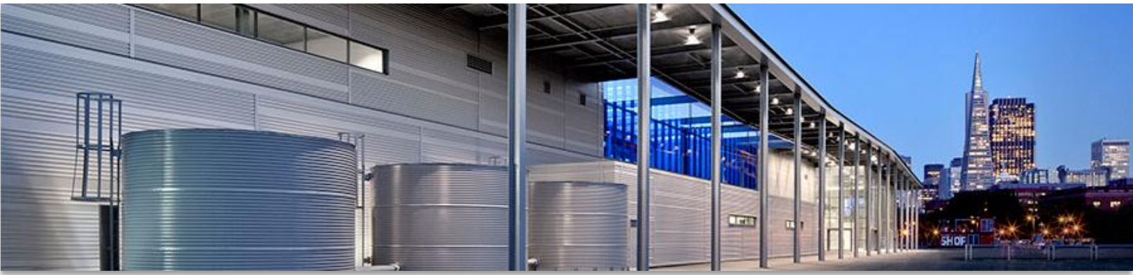
Pier 27's rainwater tanks in San Francisco, CA [Photo credit: Port of San Francisco]
