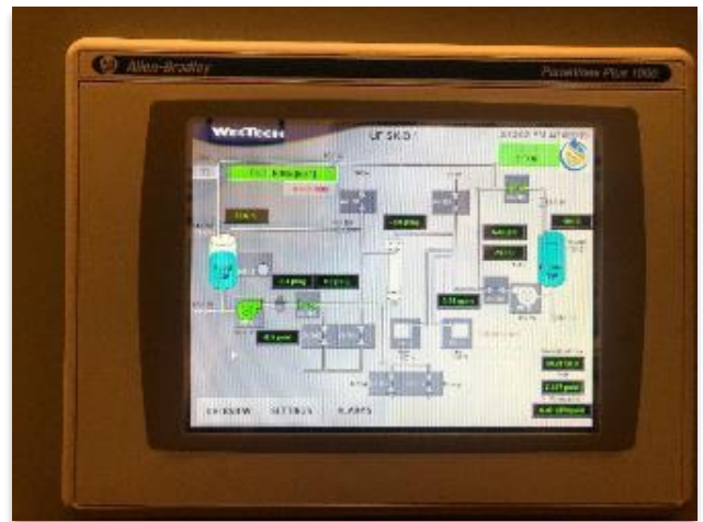
FIGURE 11.2: Operators use process control systems to access information on the treatment system in real time [Photo credit: San Francisco Public Utilities Commission. Permission to use.]
