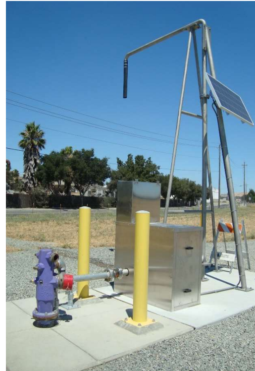
One of Central San's purple hydrants (left) and a portable meter (middle) that contractors can use to obtain Central San's recycled water. Central San's Commercial Fill Station (right).
