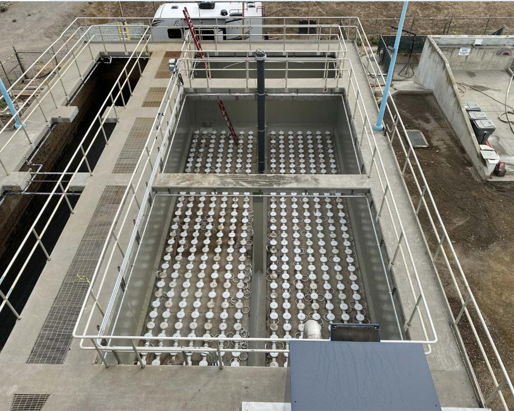
*Oro Loma Sanitary District installed of a full-scale Microvi wastewater side-stream treatment system to treat nutrients at their treatment plant in San Lorenzo, CA. The innovative watershed nutrient permit for SF bay facilitated the evaluation and select*
