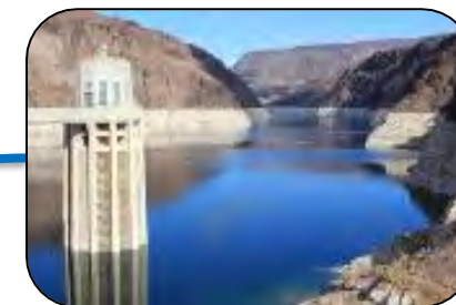
Colorado River Aqueduct
