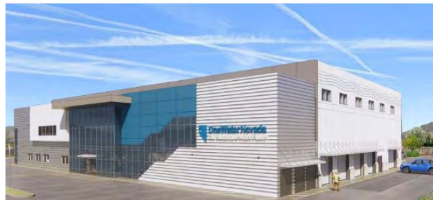
OneWater Nevada Program
