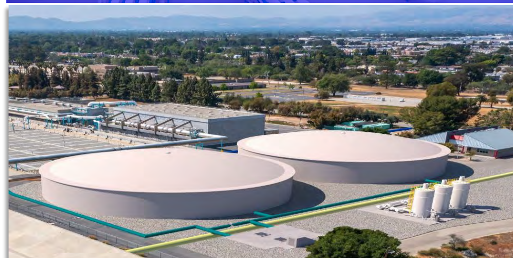
EQUILIZATION TANKS (8 MG STORAGE)
