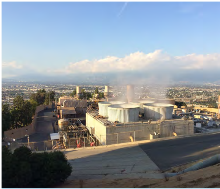
Puente Hills Gas-to-Energy Facility (Whittier)
