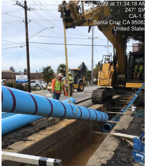
Dual 16" Pipe Installation
