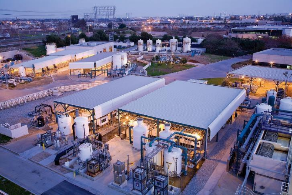
Edward C. Little Water Recycling Facility El Segundo, Calif.
