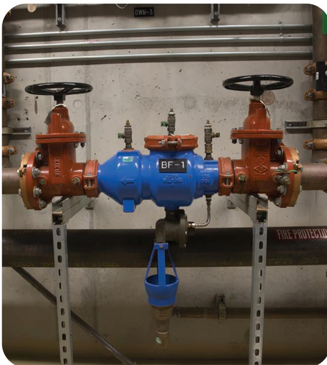
Properties that have onsite water reuse systems must include a containment reduced pressure principle backflow prevention assembly located as close as practical to, but in any case within 25 feet downstream of the point of connection to the public water system or water meter, and an air gap at the point of potable make-up to the non-potable system.
