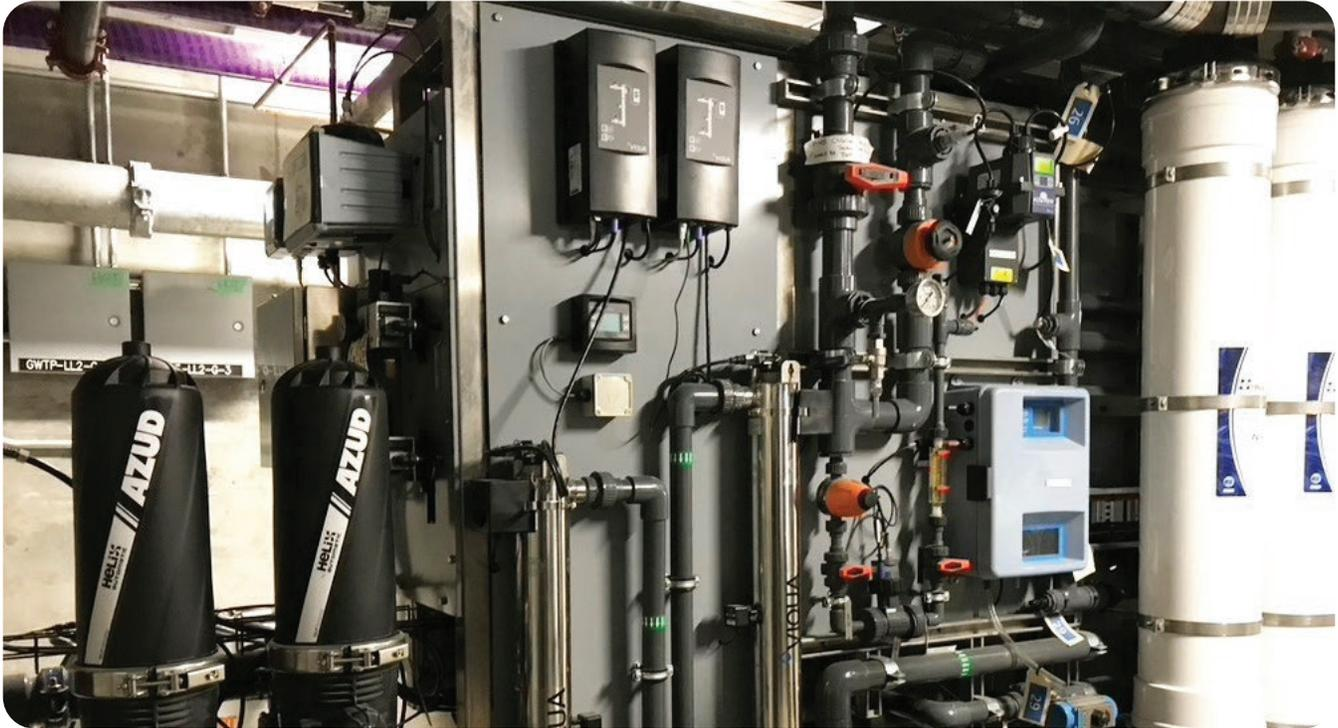
Chase Center, the sports and entertainment complex in San Francisco's Mission Bay neighborhood, is designed to collect and treat rainwater, stormwater, graywater, and condensate to supply toilet flushing demands in the arena and two accompanying office buildings.
