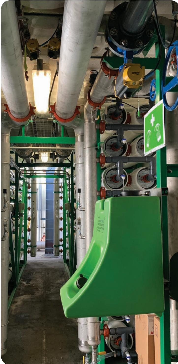
Energy Center San Francisco captures foundation drainage from Powell Street station and redirects it to their District Energy Plant nearby for producing steam. The plant has an eye wash station for the safety of all personnel working on the onsite treatment system.
