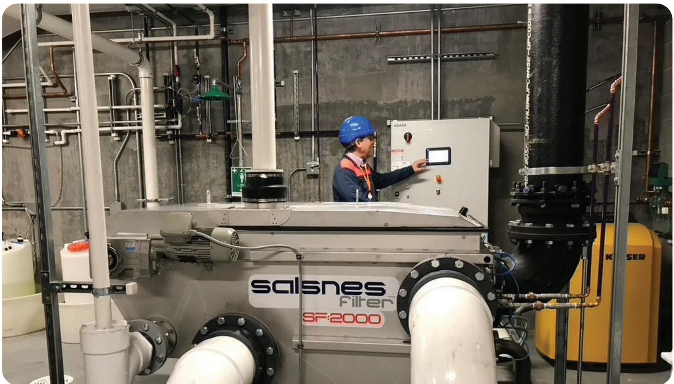
In the basement of the Salesforce Tower, the building has an onsite blackwater system that is designed to capture all of the building's wastewater, treat, and reuse it for toilet flushing and drip irrigation.
