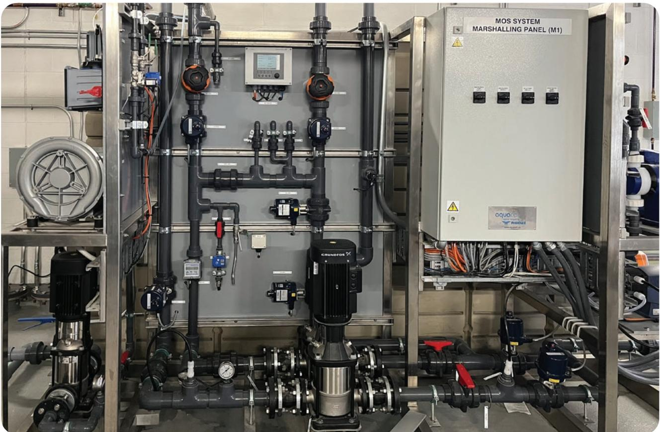
Mission Rock's district-scale blackwater treatment system is the first of its kind in San Francisco. The system will meet all of the demands for toilet and urinal flushing and irrigation and is estimated to offset about 55% of the development's total water demand.
