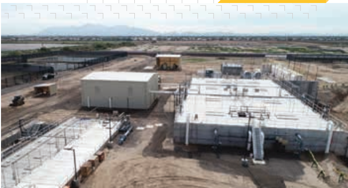
Luke 303 Water Reclamation Facility Phase 1 Expansion, Progressive Design-Build | Litchfield Park, AZ
