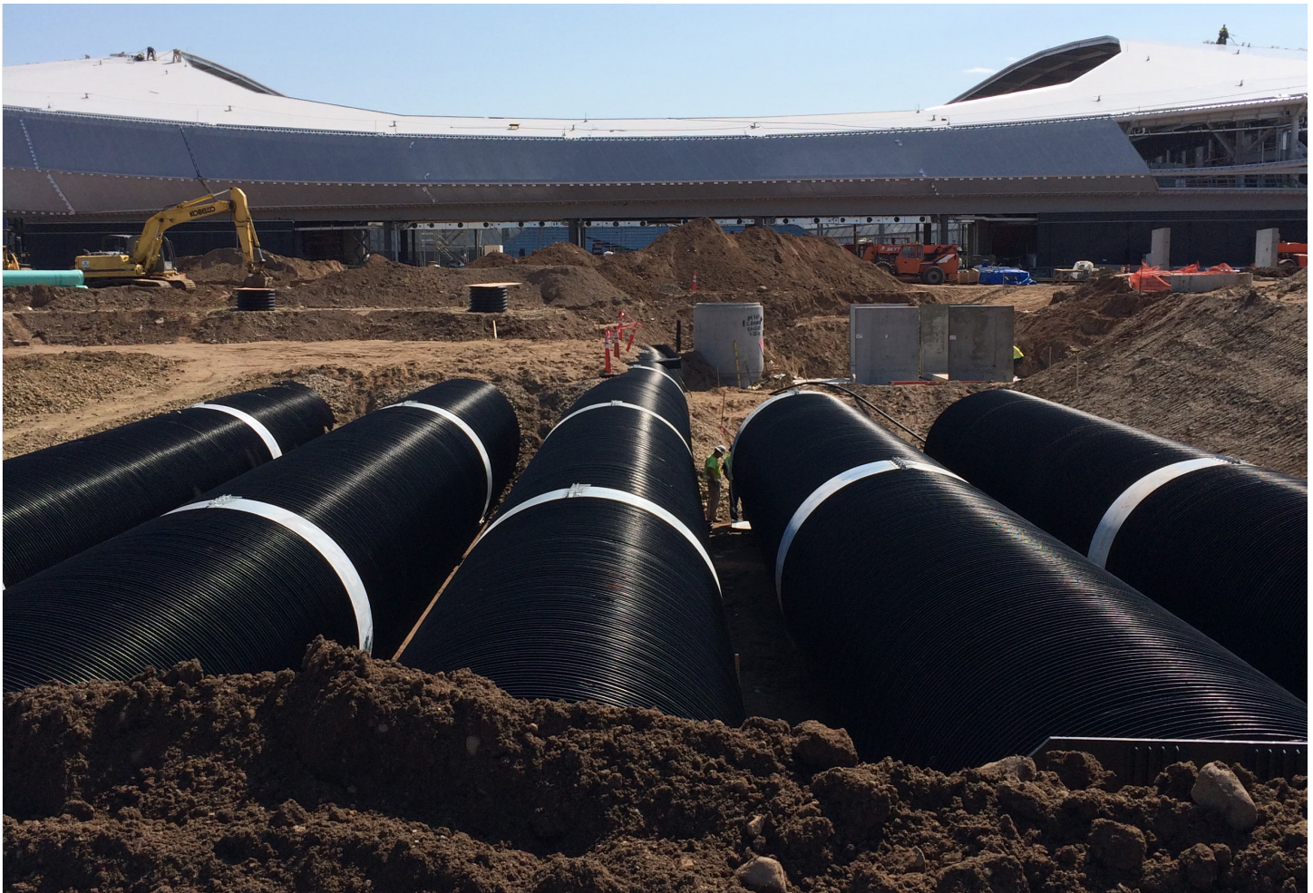
Installation of Underground Rainwater Storage Tank for irrigation of Allianz Field in St. Paul, MN (image courtesy of City of St. Paul).
