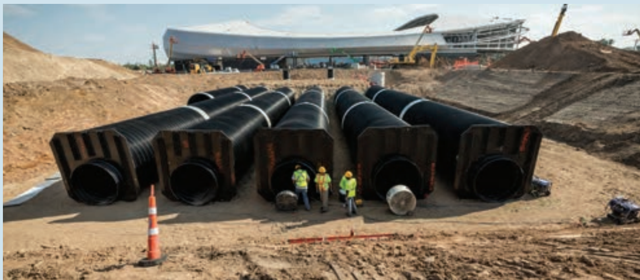
Installation of Underground Rainwater Storage Tank at Allianz Field in St. Paul, MN (image courtesy of City of St. Paul)
