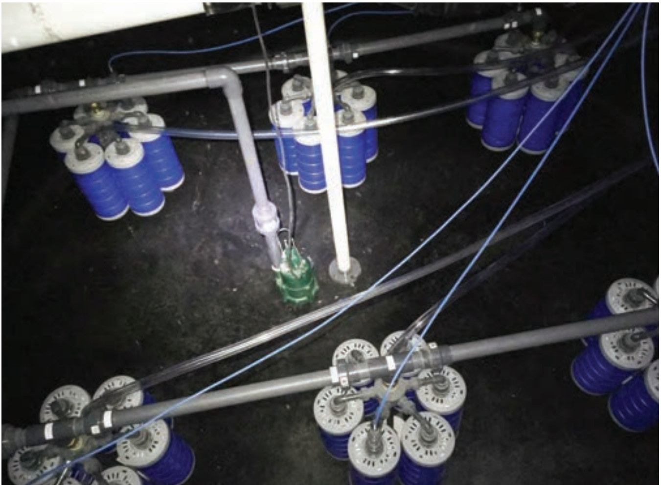
Onsite reuse system's filter cartridges (image courtesy of HTEC)
