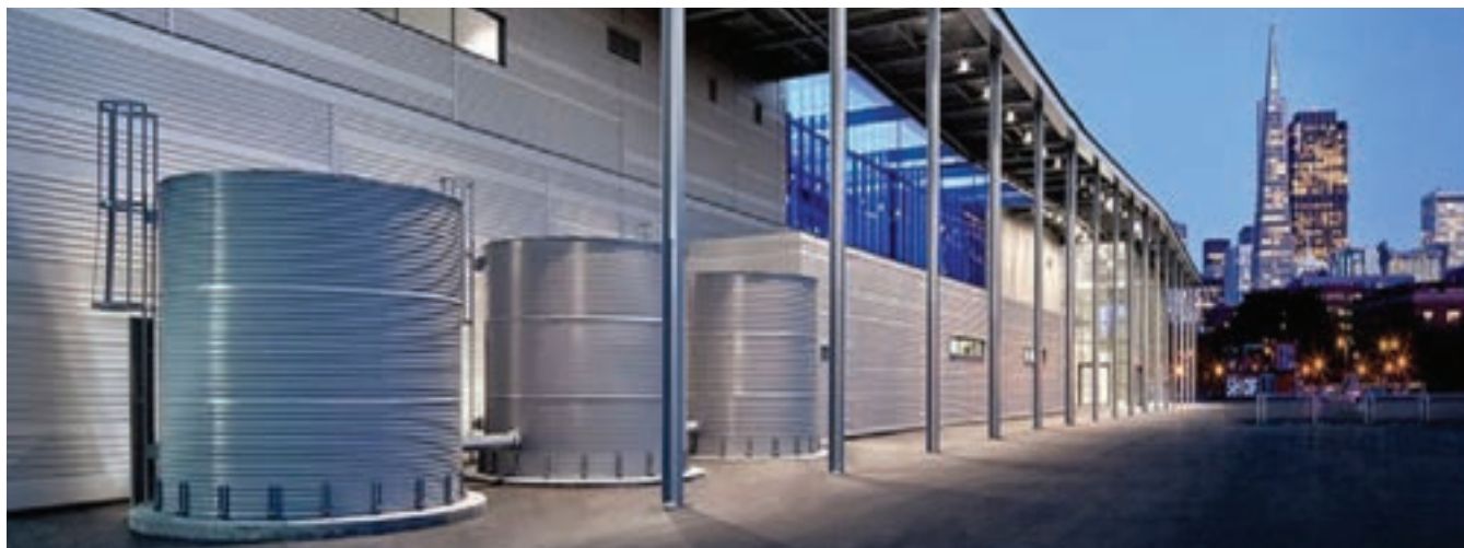
The rainwater cisterns at Pier 27 (image courtesy of San Francisco Public Works)
