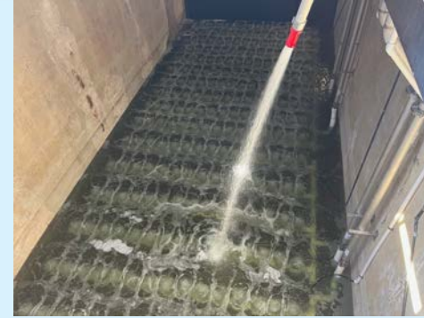
Aeration Basin Improvements - 2022
