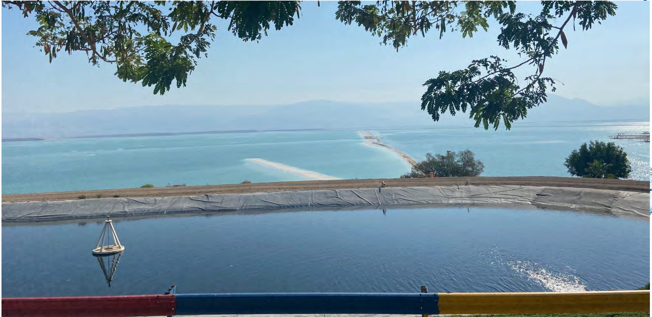
Recycled Water Storage Pond overlooking the Dead Sea
