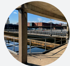
Secondary Settling Tank Refurbishment
