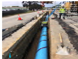
Pipeline Installation in Santa Cruz, Live Oak, Soquel, Capitola, Aptos
