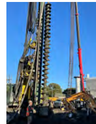
Treatment Facilities Construction in Santa Cruz and Live Oak
