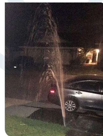
A faulty sprinkler sprays water on the sidewalk.
