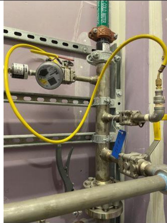
Photo 5 TLP #3 potable water PRV located on floor 6 (floors 1-7)
