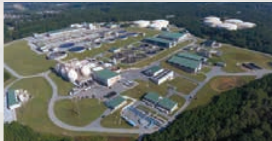
F. Wayne Hill Water Resources Center, Gwinnett County, GA
