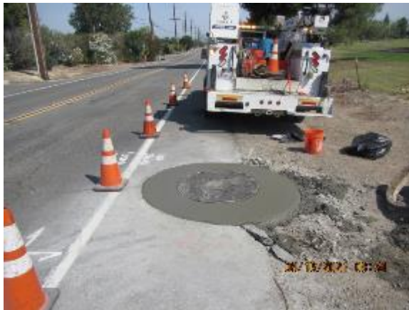
Maintenance access structure inspections and repairs
