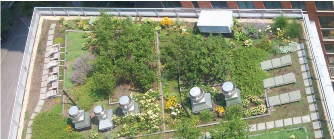
The green roof reduces runoff, insulates the building, and is irrigated by the onsite reuse system (image courtesy of NSU)
