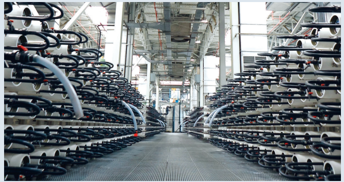
A look at the Orange County Water District's reverse osmosis (RO) facility that houses 21 RO units and 3,150 pressure vessels treating 100 million gallons of water per day.
