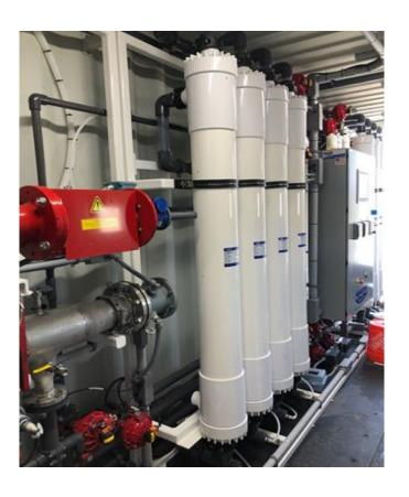
Desalitech has estimated up to 95% recovery, compared to PWR PDR estimate of 92.5% First Stage 85%, second stage 50%
