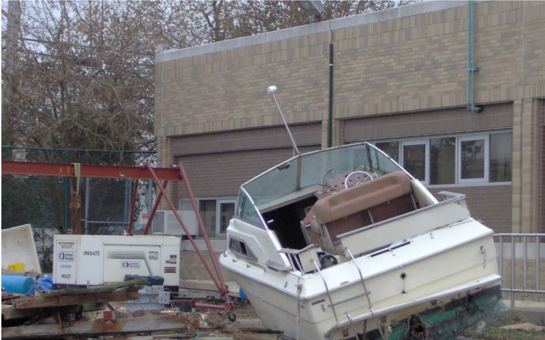
October 2012: A boat washed onto the premises of the Coney Island WWTP after Superstorm Sandy, Brooklyn, NY
