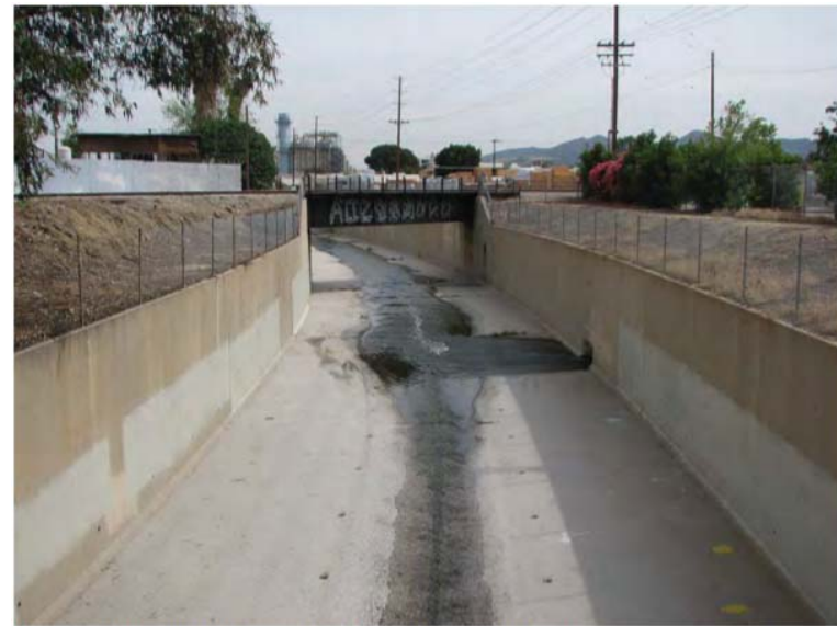
PHOTOGRAPH 1. BWRP Discharge Point 002 into a concrete-lined rectangular open channel looking downstream to the southeast.
