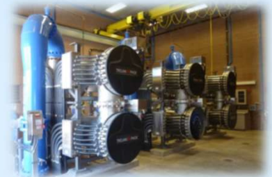
Advanced Oxidation Process (UV-H 2 O 2 )
