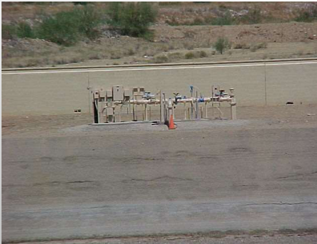
Arrowhead Water Reclamation Facility ASR Well
