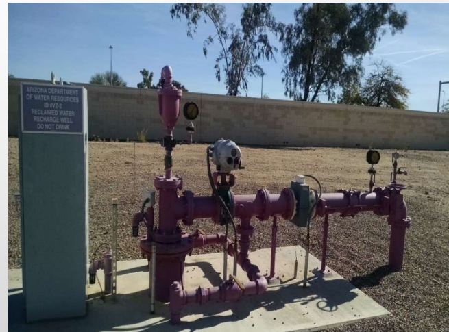
Arrowhead Water Reclamation Facility Vadose Zone Well
