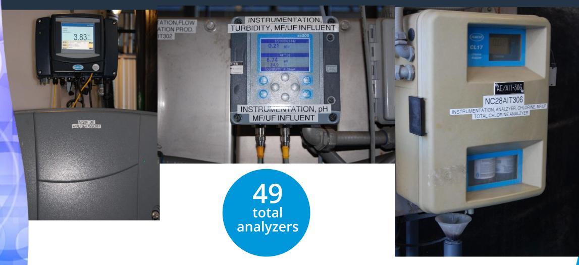
Highly reliant on instrumentation to ensure that unit processes are in the correct operating range
