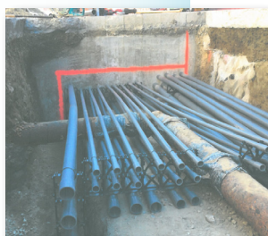
Congested ductbank and pipeline routing on a tight site.
