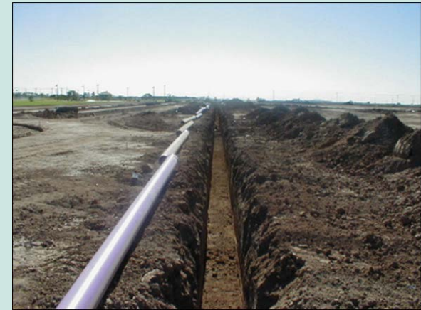
Reclaimed water pipeline, City of Chandler
