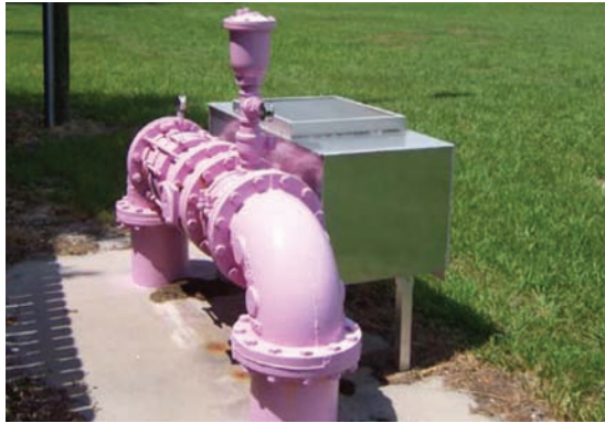
SOLAR-POWERED RECLAIMED WATER CONTROL VALVE
