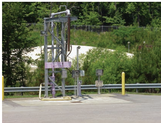
BULK RECLAIMED WATER FILLING STATION
