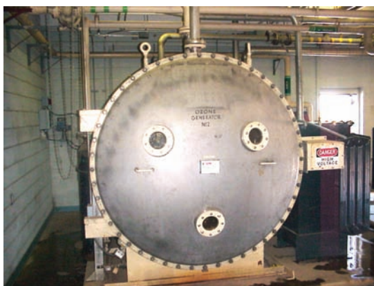
OZONE GENERATOR FOR DISINFECTION
