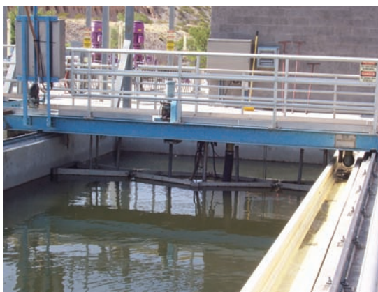
AUTOMATIC BACKWASH FILTERS
