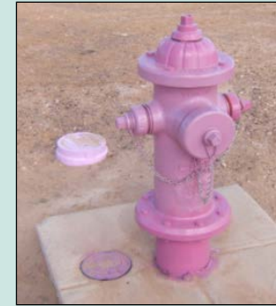
Reclaimed Water Fire Hydrant
