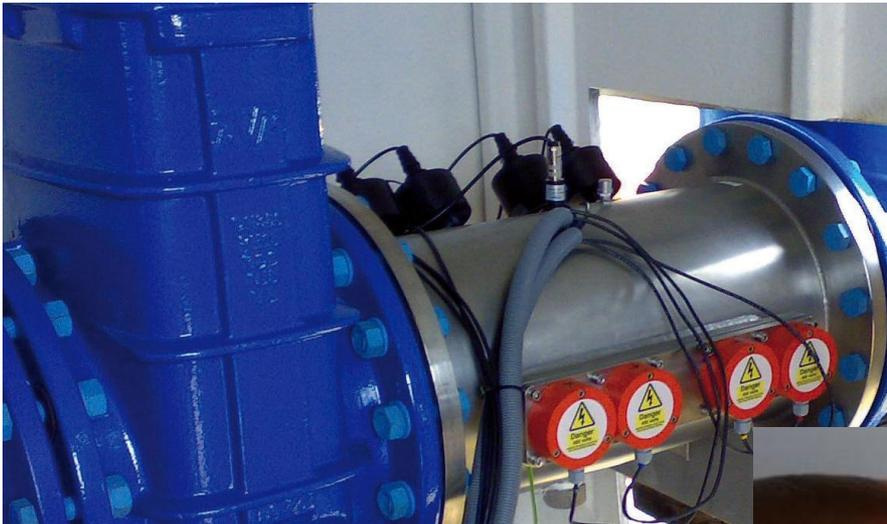
Allows for replacement of monitors and reference monitor checks without having to close valves and drain the reactor.
