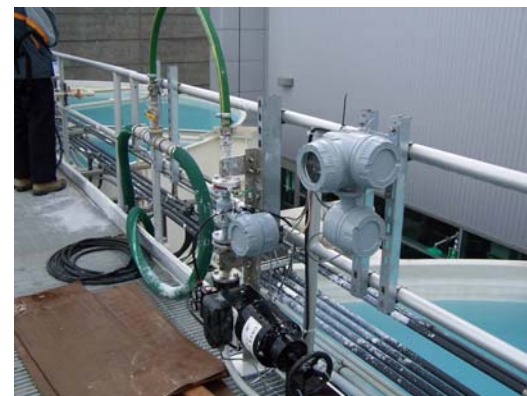
Lime Slurry Feed Assembly
