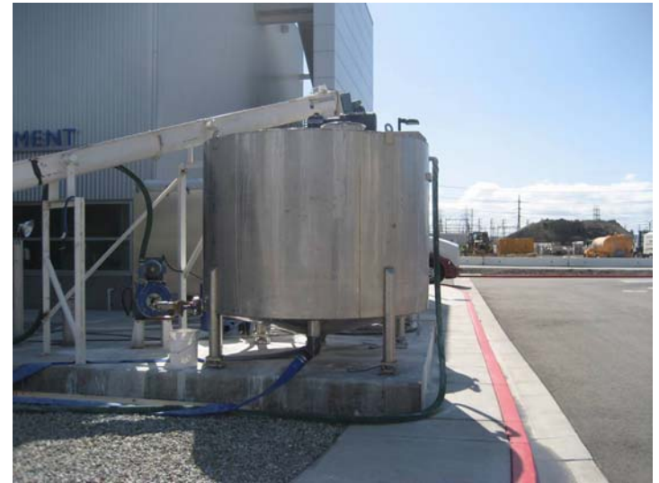
Lime Slurry Aging Tank
