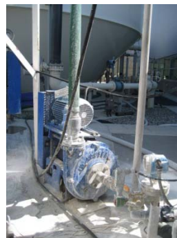
Slurry Transfer and Feed Pump
