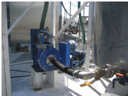
Slurry Transfer and Feed Pump
