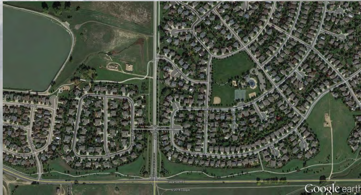
Aerial view of landscaped rights-of-way in Erie (Arapahoe Ridge)
