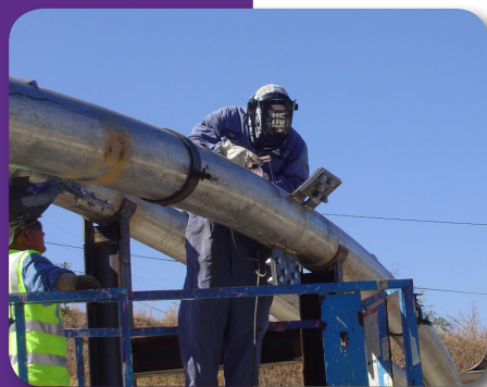
Temporary plates, braces, and supports help to fit up the mid-span weld of the crossed arches pipe bridge.
