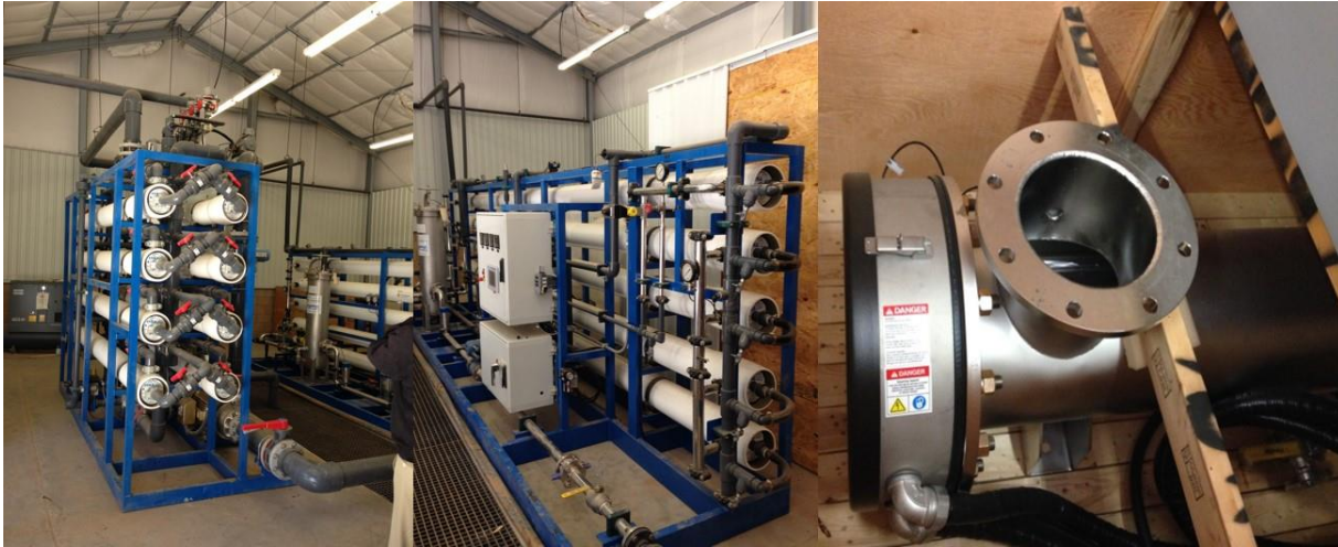
Figure 9 Cloudcroft DPR Treatment Plant (UF, RO, and UV AOP Processes) under Construction
