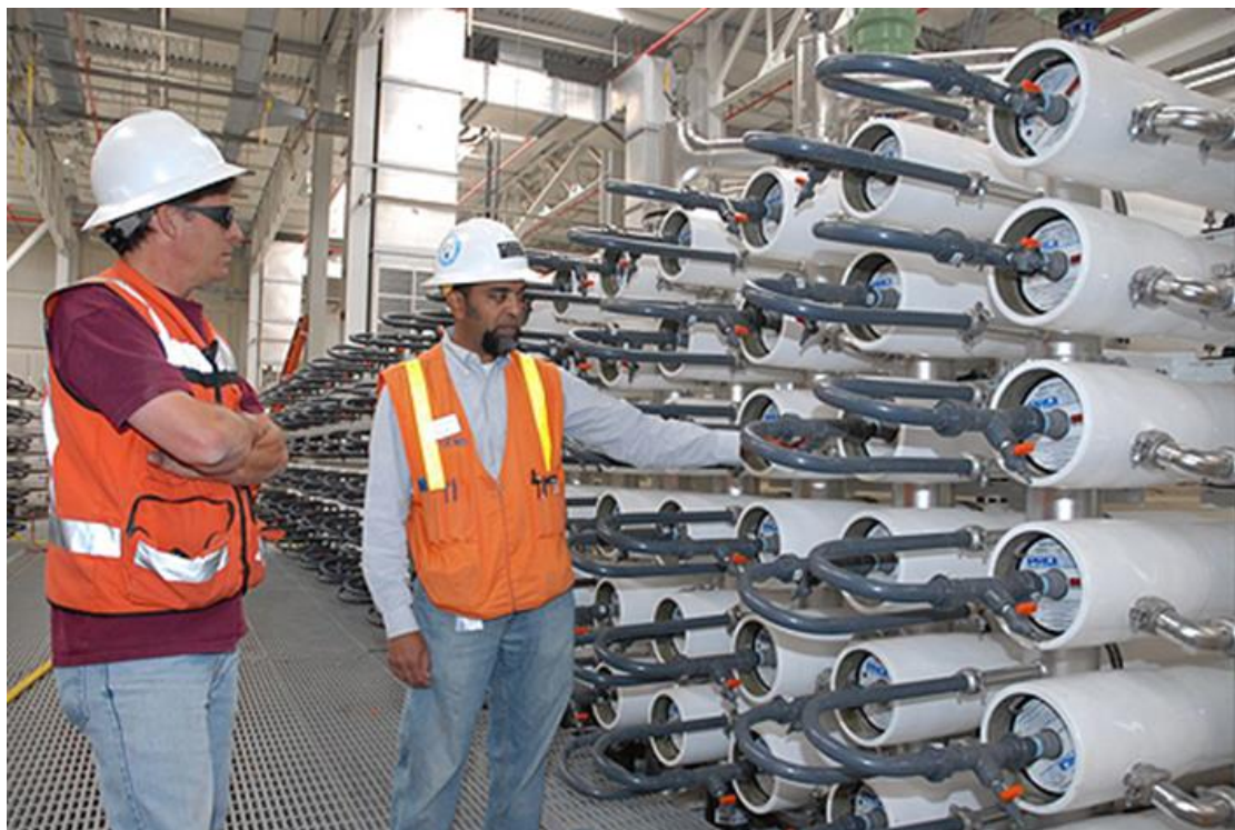
Figure 11 OCWD GWRS RO Membranes Used to Purify Reclaimed Water for Potable Reuse
