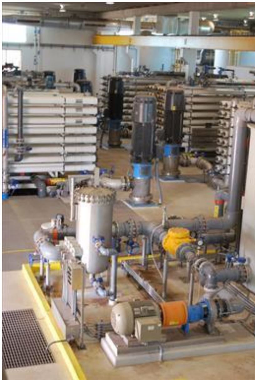
Figure 7 RO System at the Cypress Hill Water Treatment Plant in Wichita Falls Texas, used for Direct Potable Reuse ( no longer in operation due to easing of drought conditions )
