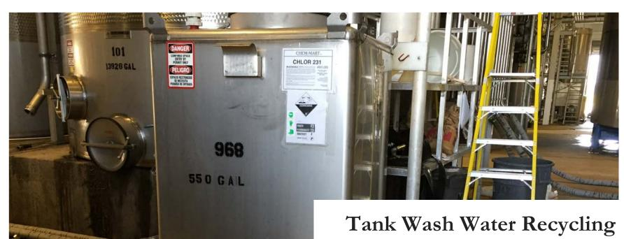
We developed a water recycling system for our stainless cellars that reuses pH balanced cleaning solution for consecutive tank washes, saving ~150 gallons of water per tank wash.
