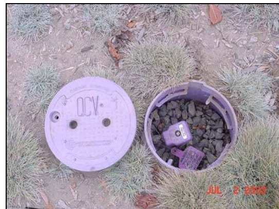
Tagged quick coupler and valve box
