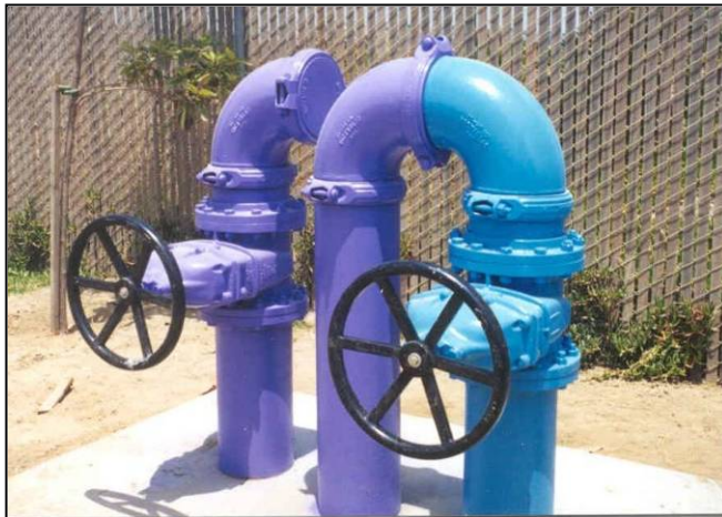
Example photos of existing "swivel-ell" assemblies for a back-up potable water supply.
