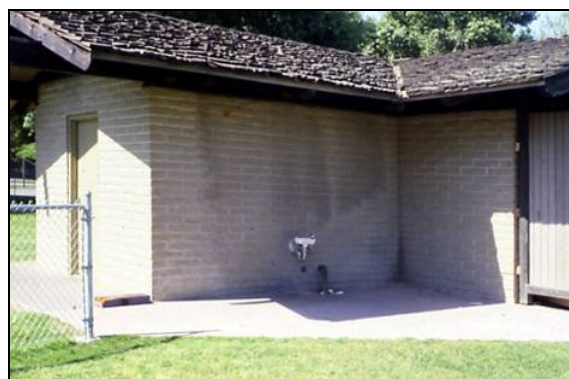
The pattern on the walls indicates that this drinking fountain is being sprayed by the irrigation water. If recycled water is to be used, then the spray pattern must be altered or the drinking fountain somehow shielded.
