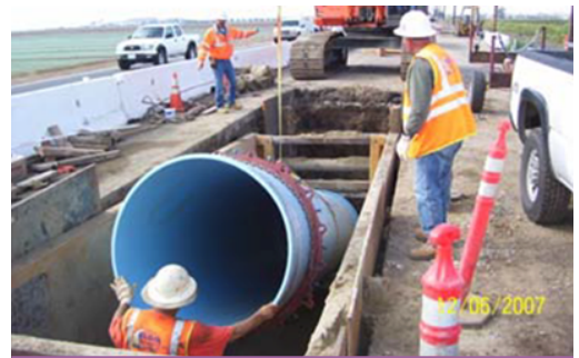
Construction of a salinity management pipeline temporarily repurposed to provide drought relief for agriculture users.
