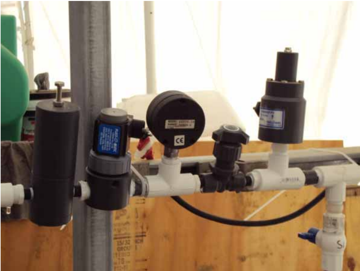
Figure 6.6. Control sequence at pilot input including pressure reducer, solenoid valve, pressure gauge, needle valve, and pressure relief valve.
