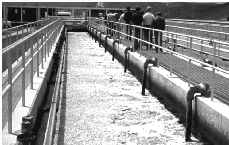
**Figure 3.2. Sample picture of an aeration tank in an activated sludge system.**
