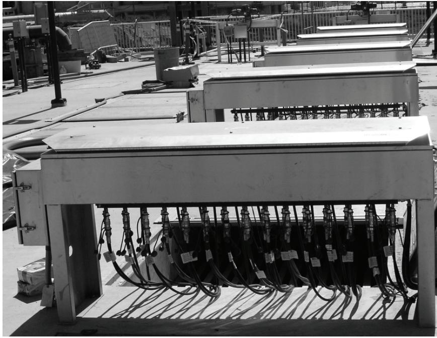
**Figure 4.5. Open-channel UV disinfection system by Trojan Technologies.**
