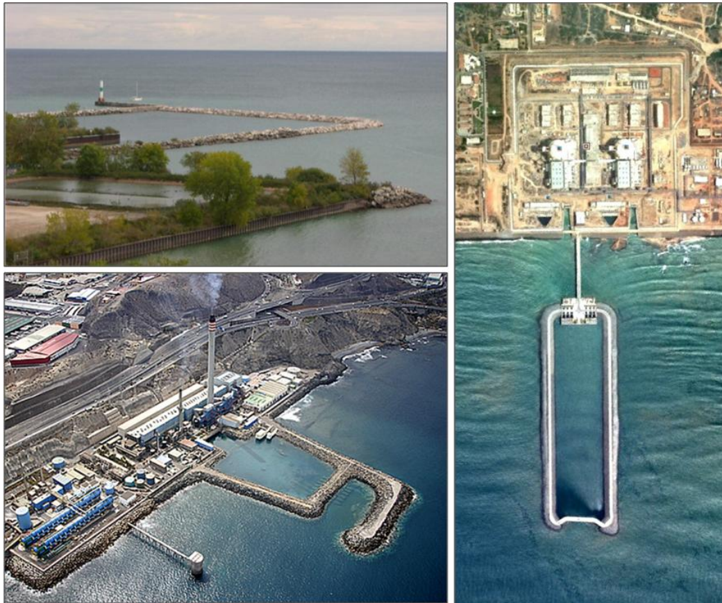
Figure 3.9. Existing porous dikes used at industrial intakes. Clockwise from top L: We Energies' Port Washington Generating Station on Lake Michigan; Kudankulam Nuclear Power Plant; Gran Canaria desalination plant.
