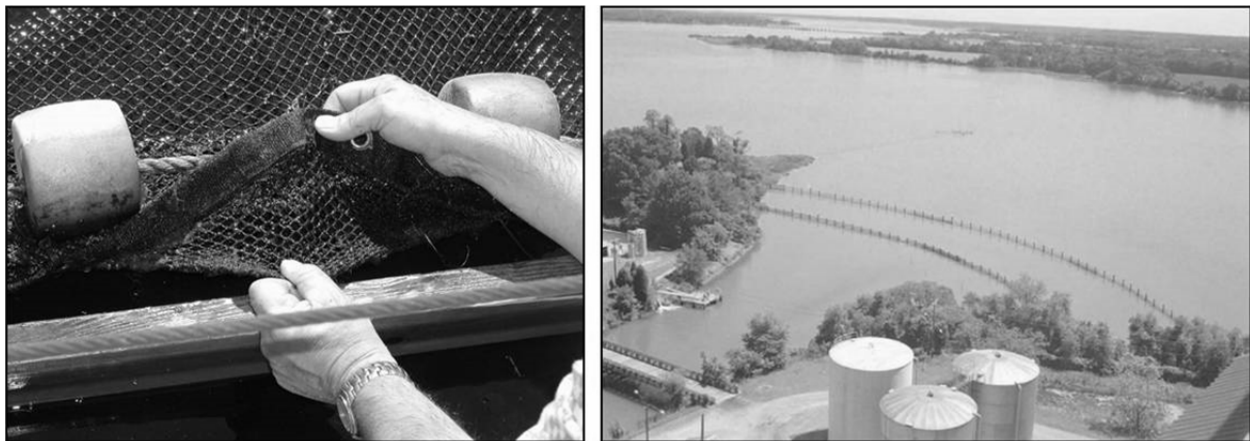
Figure 3.8. Barrier net mesh (L) and barrier net system (R) at Chalk Point Generating Station on the Patuxent River, MD.
