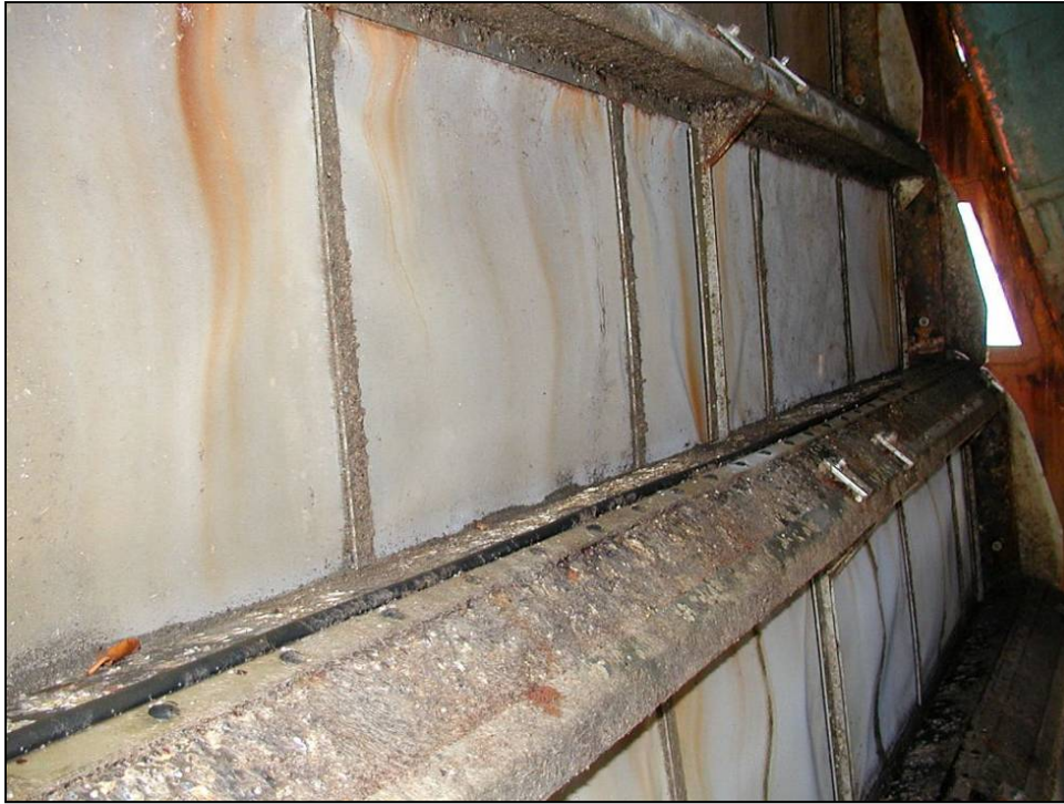
Figure 8.6. Fine-mesh screen panel at Big Bend.
