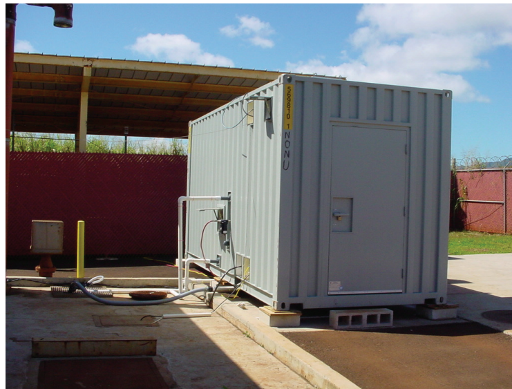
Figure 2.6. Containerized Zenon pilot MBR at a pump station in Wahiawa, HI.
