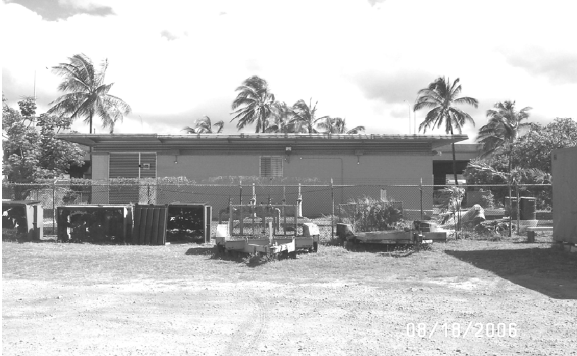
Kamehameha Highway Wastewater Pump Station. This pump station is a potential wastewater source for an MBR facility that could provide recycled water to Keehi Lagoon Park and the HIA. Nimitz Highway and the H1 Viaduct, behind the pump station building in this photograph, are north of the pump station.
