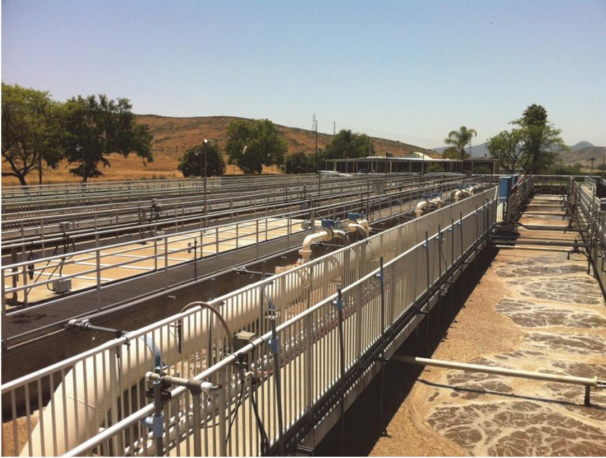
**Figure 2.23. Padre Dam WRF's secondary treatment aeration basin (first aerobic stage).**
