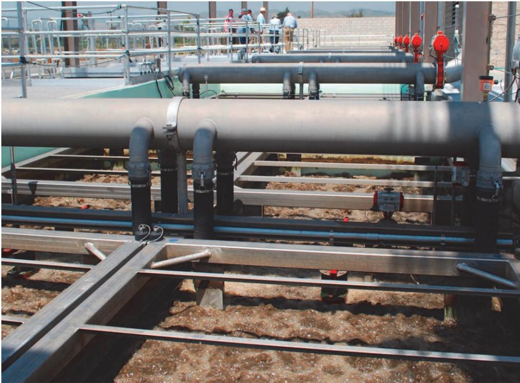
**Figure 2.10. Santa Paula WRF's membrane separation tanks.**
