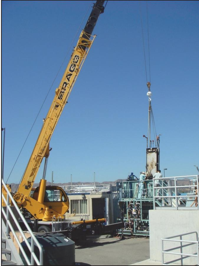
**Figure 6.6. Uninstalling the membrane module to breach the membrane.**
