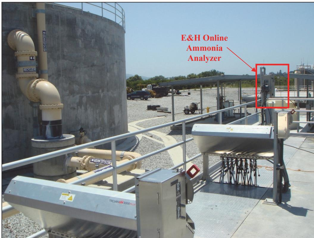
**Figure 3.9. Online ammonia analyzer installed at the CA-01 facility.**
