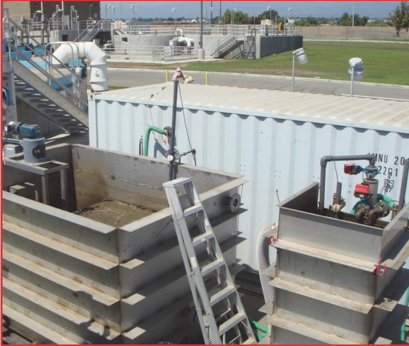
**Figure 3.6. Photograph of MBR Pilot System B.**
