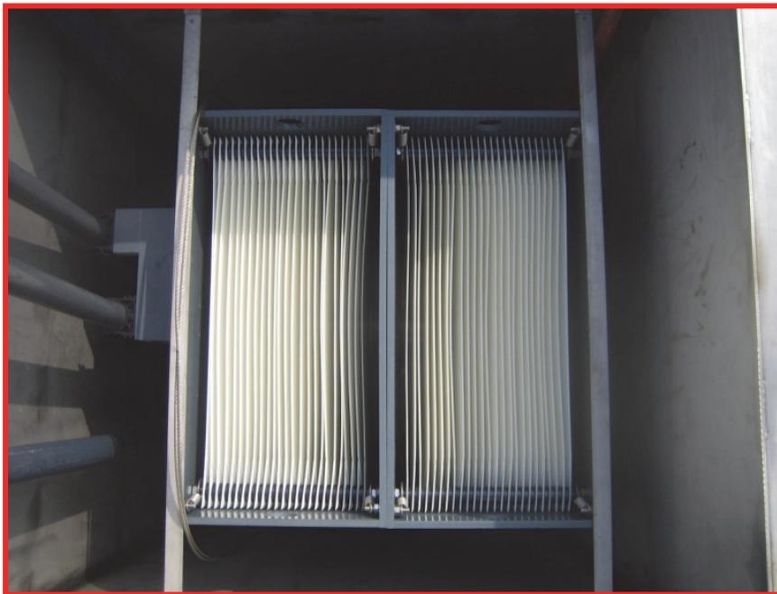
**Figure 3.7. Photograph (top view) of the Pilot System B membrane module.**
