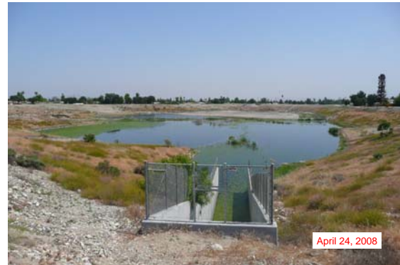
Figure 2.19. View of IEUA's 8th St. Basin's surface spreading operation.
