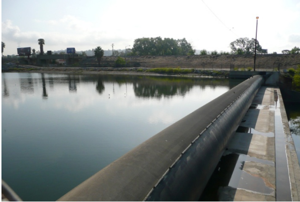
Figure 2.3. Rubber dam in the San Gabriel River.
