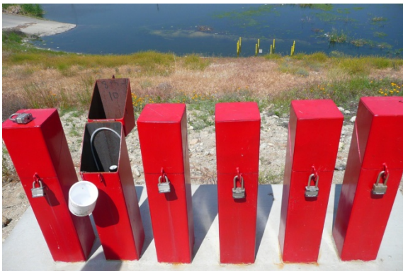
Figure 2.20. 8th St. Basin's lysimeter sampling ports.
