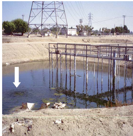
Figure 2.7. Close-up of USGS/WRD test basin, catwalk access to sampling points. Arrow indicates location of reclaimed water inlet.
