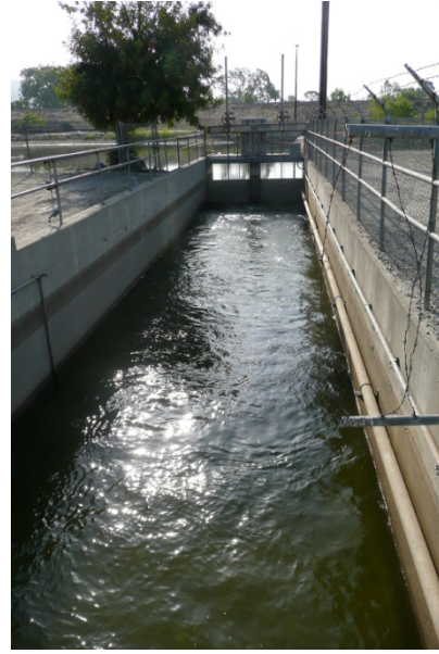
Figure 2.4. Intake structure for the SGCB.
