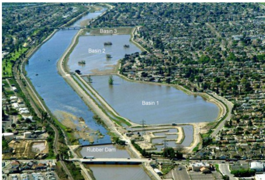
Figure 2.1. San Gabriel Coastal Spreading Grounds.
