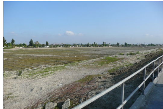
Figure 2.2. Dried recharge basin at SGCB.
