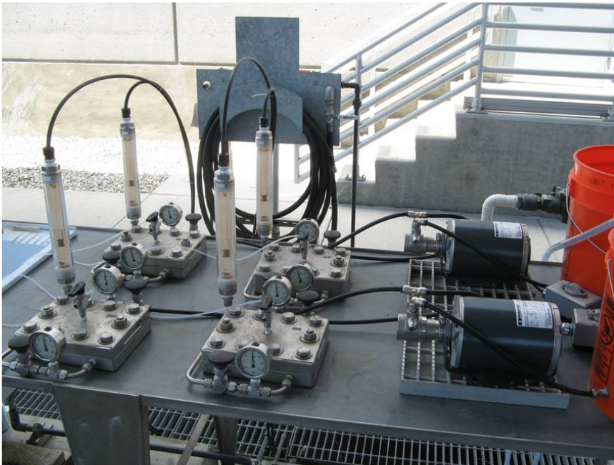
Figure 4.41. RO flat sheet test cells.
