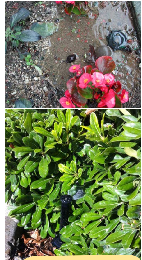
Some of the most common causes of poor irrigation performance are irrigation heads that are broken (top) or obstructed by large shrubs (bottom).
